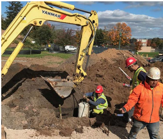
Lighting system being installed. Connections have also been made to the proposed solar array site with the building.
