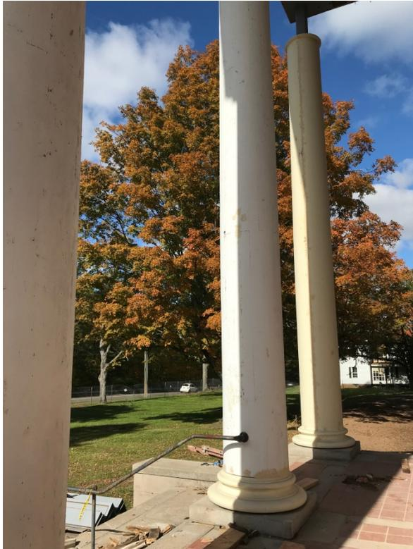
Three columns on the westerly portico facing Eastern Drive being prepared. The column furthest to the right is a replacement column with new steel inside the column.
